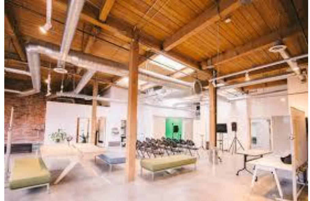
New Concrete Floors Creating Structural Diaphragm
