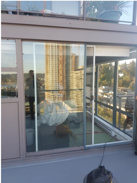
Glazing being reinstalled to frames
