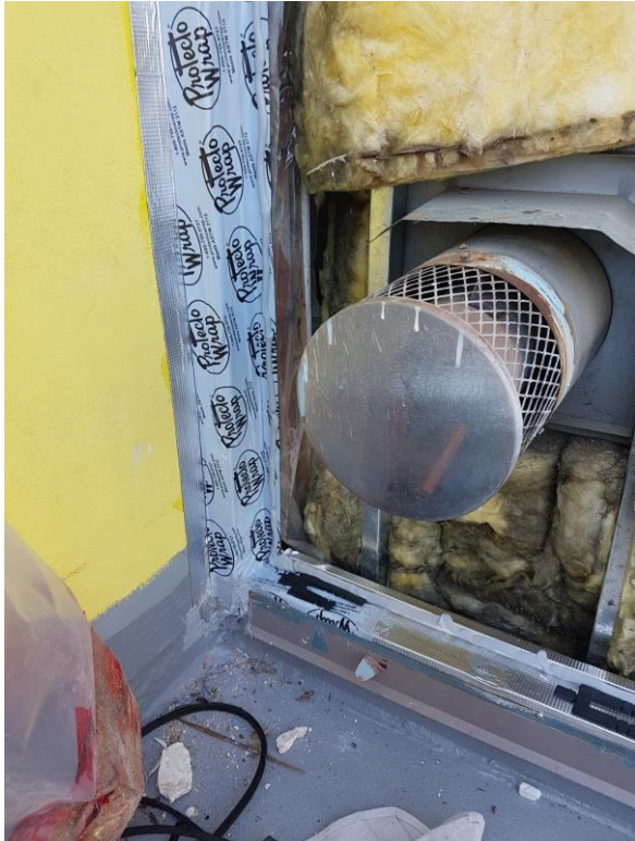
Prep for frame to be installed
