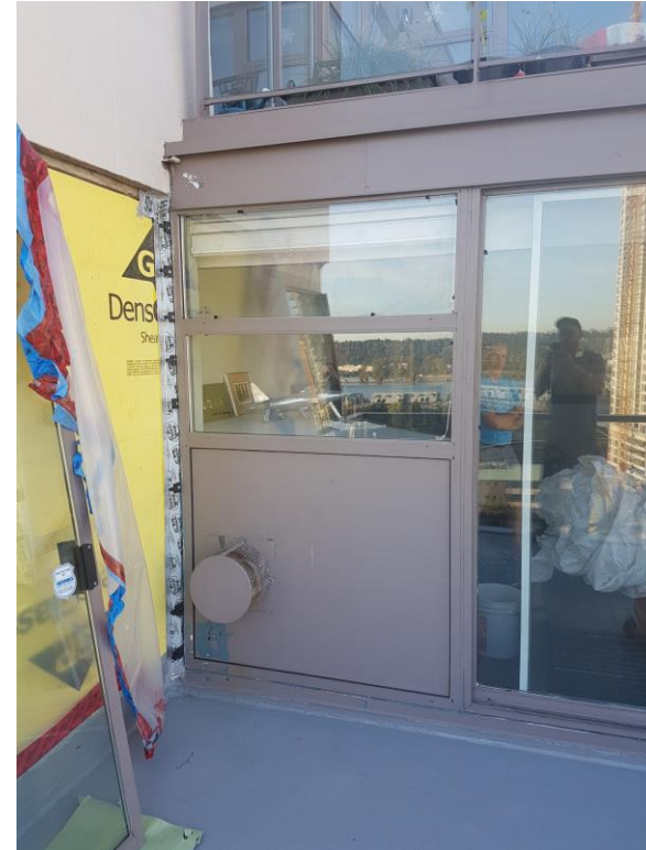
Frame being reinstalled
