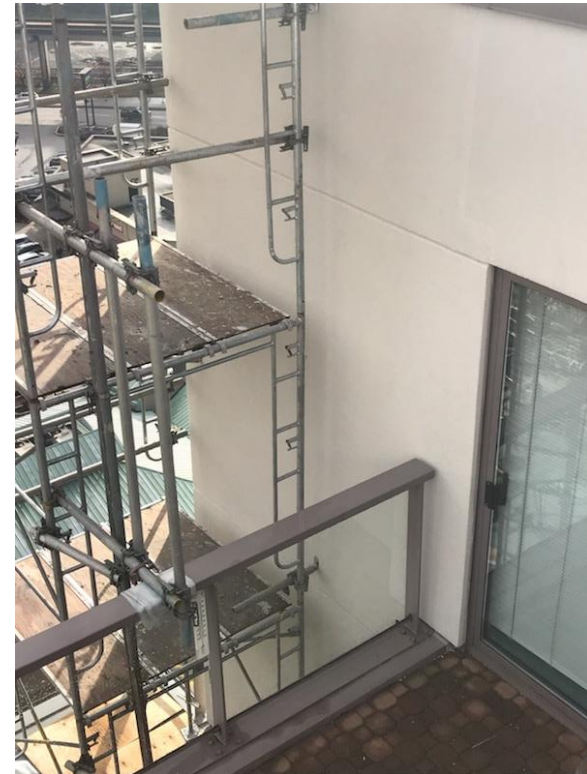
Scaffolding For Stucco And Painting
