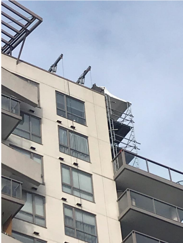
Swing Stage and Weather Protection
