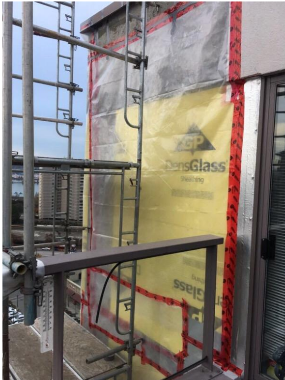
Stripping Damaged Stucco Assembly
