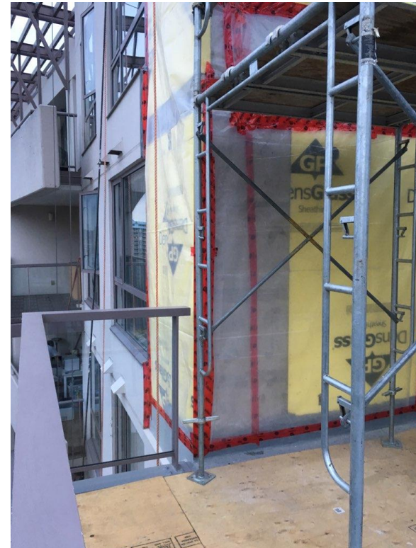
Scaffold And Temporary Protection
