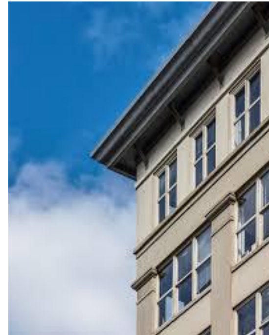
New Cornice Added
