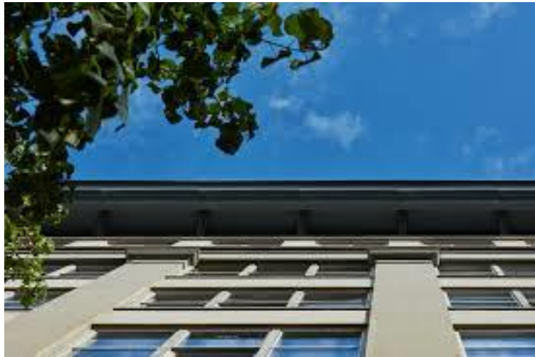
New Cornice and Windows
